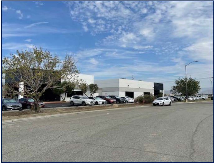
Photo of the industrial building with an adjacent building
