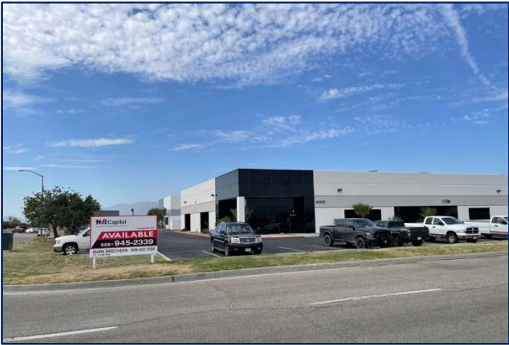
Photo of the subject site industrial building view from Avenue 54. Suite H is located at the corner Suite.
